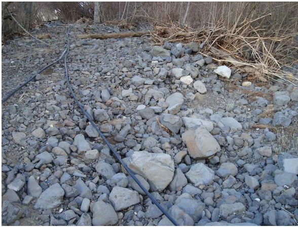
The previous creekbed, now full of rock pushed downstream by flood waters.
